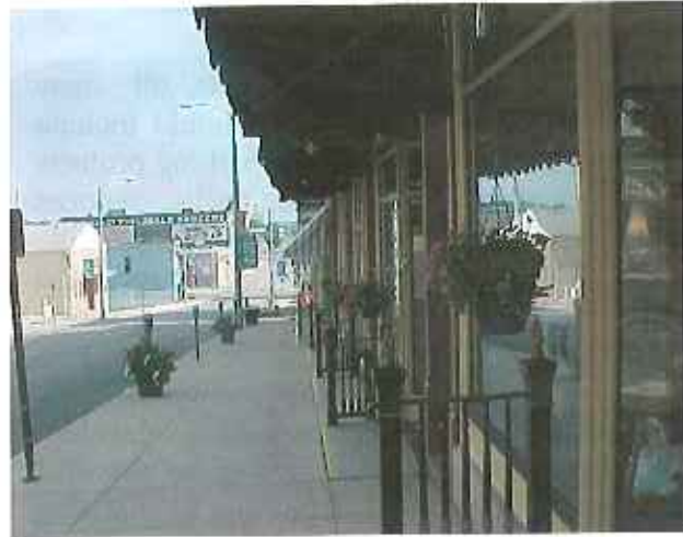
Mansfield, Ohio Storefront renovation
